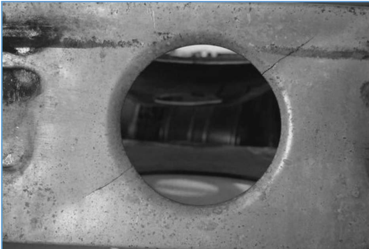
Figure 1 Crack in the Center Lightning Hole on the Horizontal Stabilizer Forward Spar (example)
